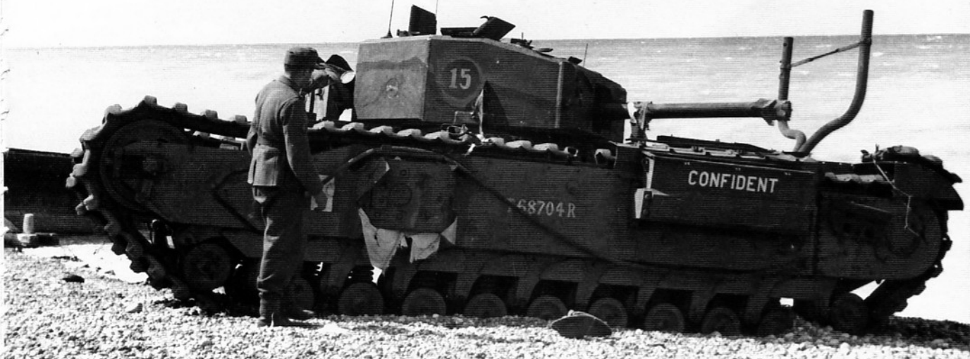
Churchil Mk. III of C Co. with air-intake lubber for action on the beach.
